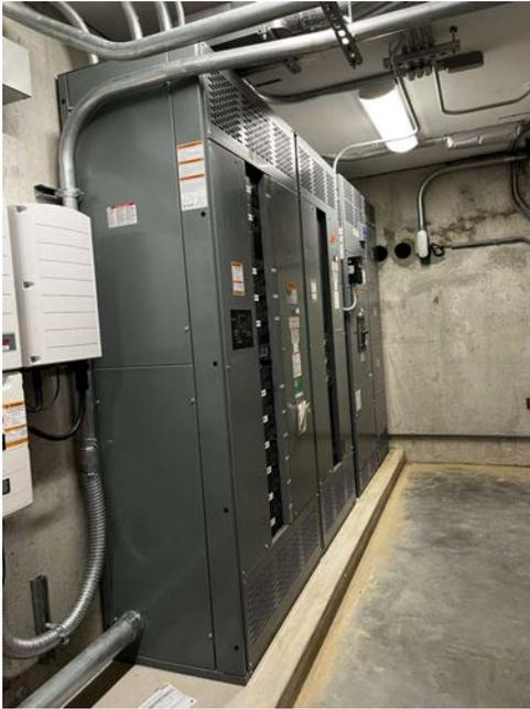
**Figure 3. Inverters and transformers for solar systems in the Horn Hall electrical room.**
