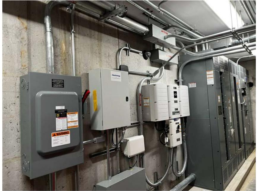
**Figure 4. A diagram of the electrical components for the rooftop solar system outside of Horn Hall.**
